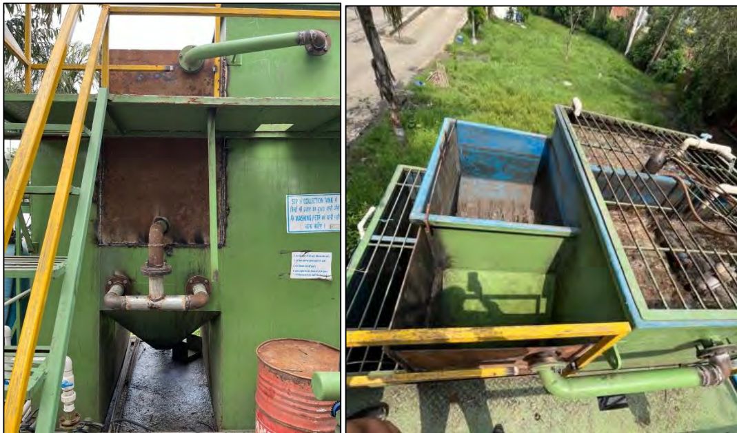
TUBE SETTLER: AFTER MODIFICATION
